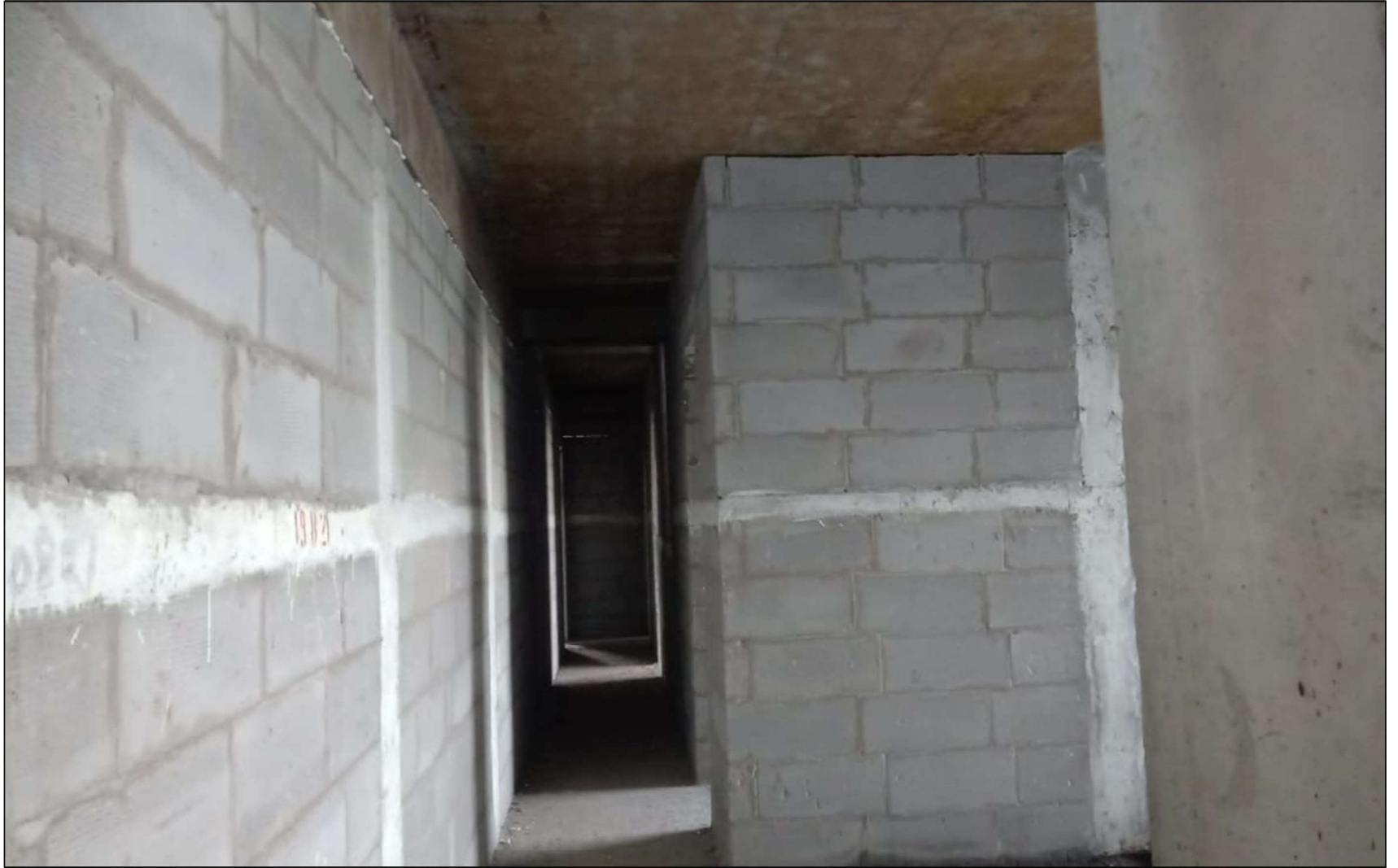
7 th Floor works under progress
